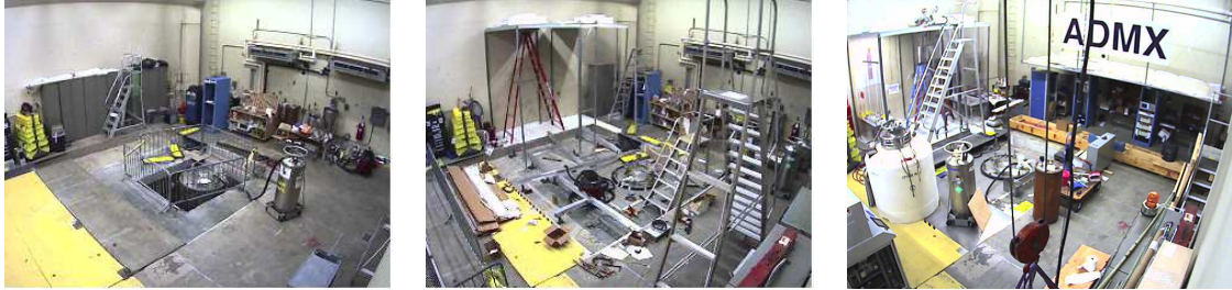
Figure 5.1-1. Progress of the ADMX experiment site at CENPA. Left : July, 2011, showing the initial magnet installation. Middle : November, 2011, showing the beginnings of flooring and clean room. Right : February, 2013, showing the clean room with experimental insert, helium-liquefaction system, and data-acquisition racks.
