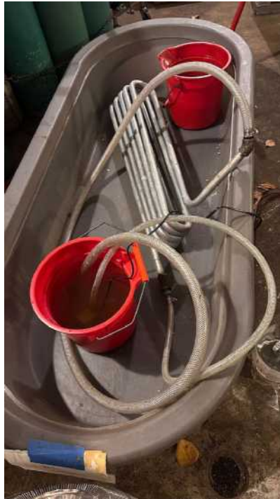
Figure 6.2-2. Newly fabricated Ingersoll-Rand coil acid flush before installation.
